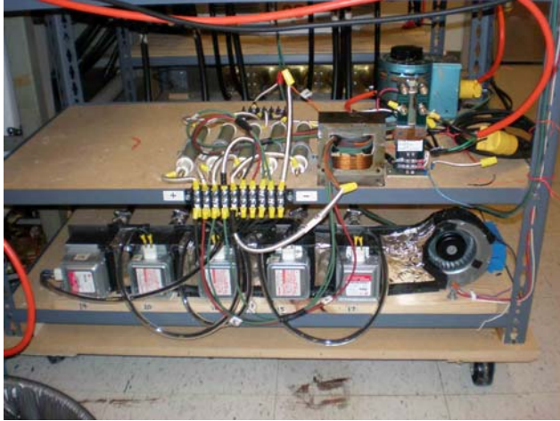
Figure 3.16: Group of five magnetrons, fan, HV relay
